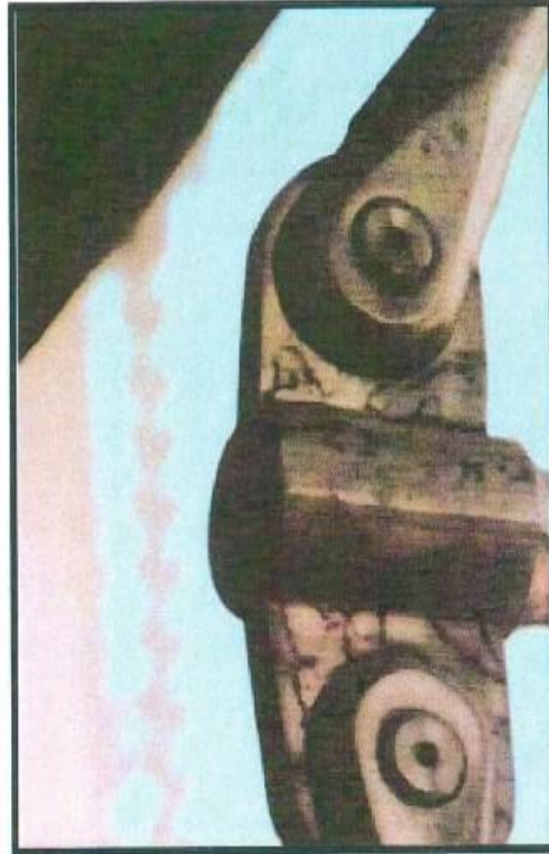
Views showing cracks within the Wind Load Steel Struts
